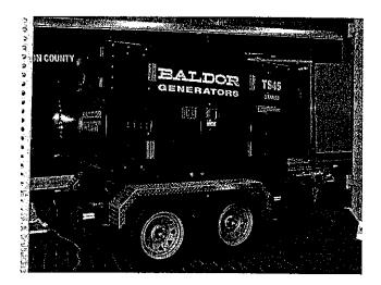
45 KW mobile generator can supply electrical needs as a stand alone unit or can be hard wired into electrical distribution system in building. Has an 80 gallon fuel capacity.
